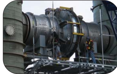
Inline Pressure Balanced Expansion Joint
