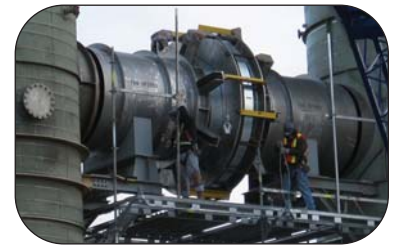
Inline Pressure Balanced Expansion Joint
