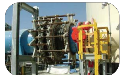
In-line pressure balanced rubber expansion joints
