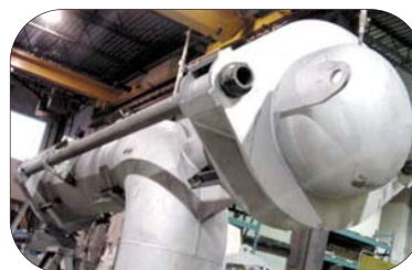
Pressure balanced crossover expansion joints
