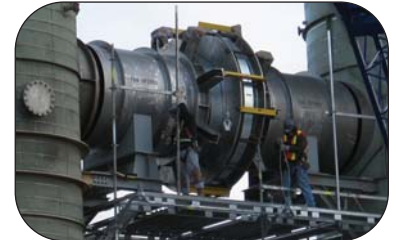
In-line Pressure Balanced Expansion Joint
