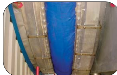
Flue Gas Corrosion Resistant Ducting Expansion Joint
