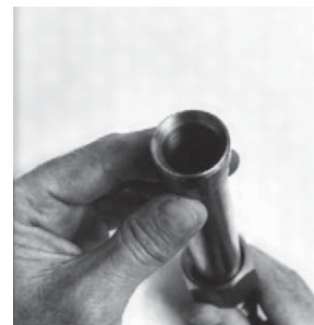
4- Inspect flare before installing
