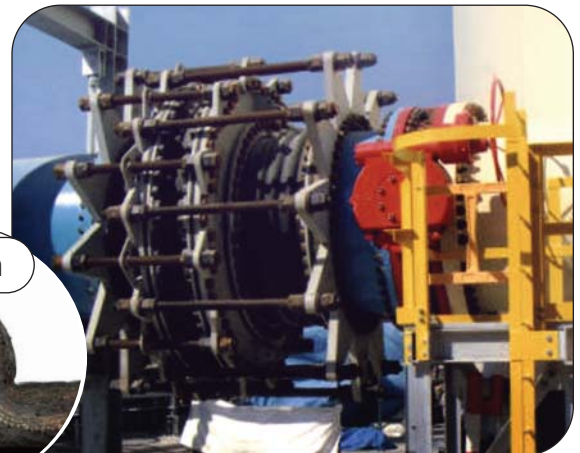
42IRPB™ with exterior coating (to protect elastomer from severe ozone radiation) installed at Saudi Petroleum in the Kingdom of Saudi Arabia
