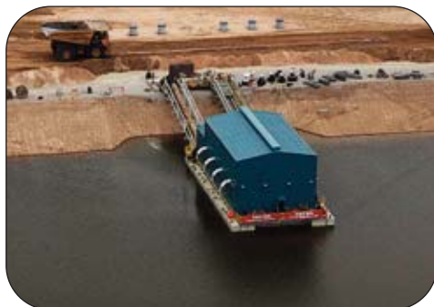
Water reclaim barge pump house in operation
