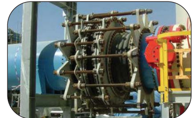
Rubber inline Pressure Balanced Expansion Joint
