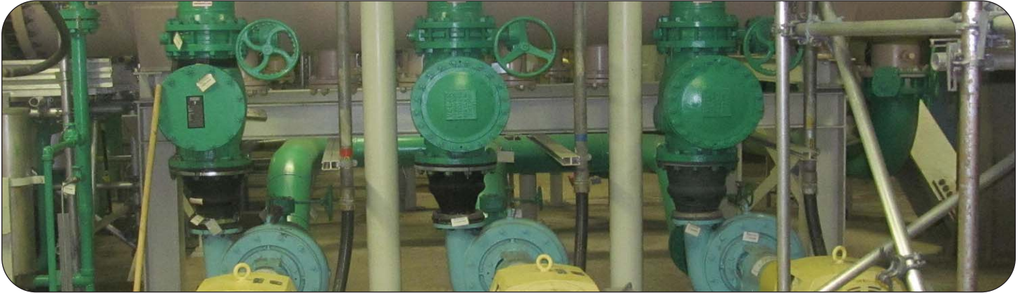
Thorburn's 42HP-CR Concentric & 42HP-OR reducing expansion joints installed in pumping station at the OPG Pickering nuclear reactor
