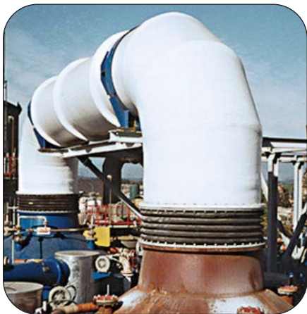
Quantity of 12 Thorburn 62HPW 900mm (36") Rubber Expansion Joints installed on a GRP piping system at a sulphuric acid plant in Baja Mexico
