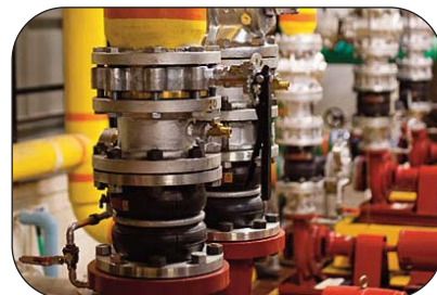
Thorburn model 201 twin sphere joints installed at a pumping station
