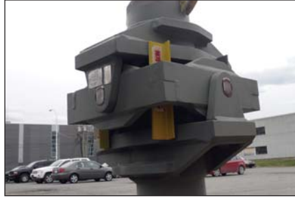
Restrained Gimbal (10,000 kPa) Expansion Joints
