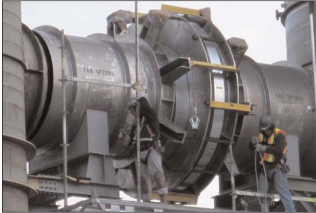
Thorburn's multi-convolution high pressure ASME SEC VIII, DIV. I Appendix 26 pressure balanced metallic bellows expansion joint is used for critical hydrocarbon processing application for Shell Canada's Blackrock Project
