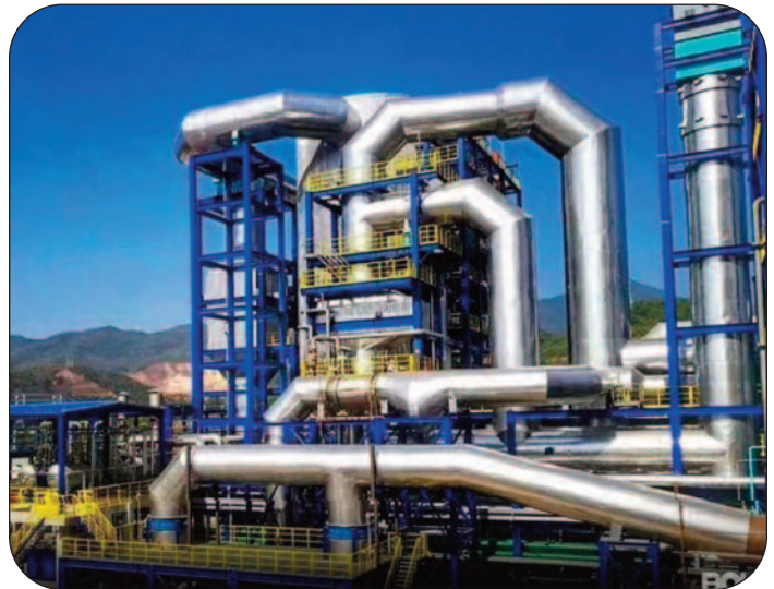
Thorburn's High-Core bellows expansion joints are used in acid plant piping systems
