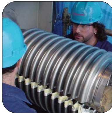
Thorburn Series CRS penetration seals were site welded together without cutting the steam pipe
