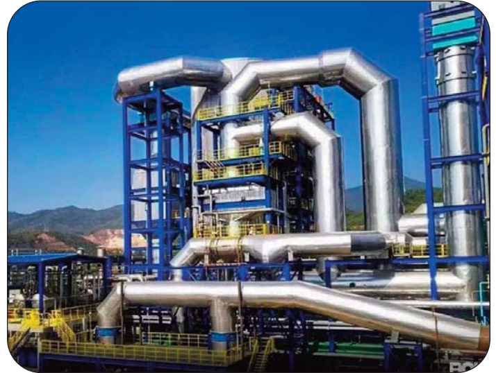
Thorburn's High-Core bellows expansion joints are used in acid plant piping systems
