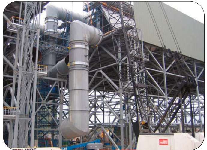
Tied double universal expansion joint
