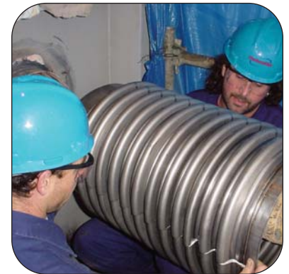
Thorburn Series CRS penetration seals were site welded together without cutting the steam pipe
