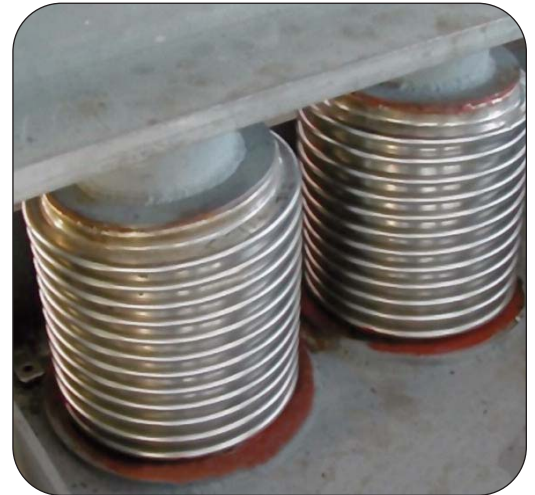
Sidewall and roof penetration seal bellows are found in HRSG power plants
