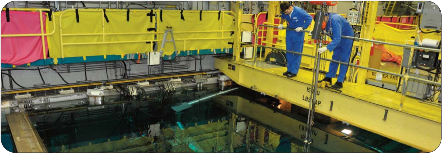
CANDU 6 spent fuel storage bay
