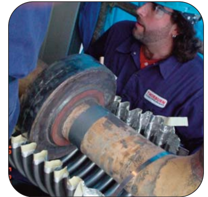
Thorburn site team replaced a failed fabric penetration seal with a series of retrofit seals
