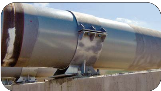
Pipe Alignment Guide
