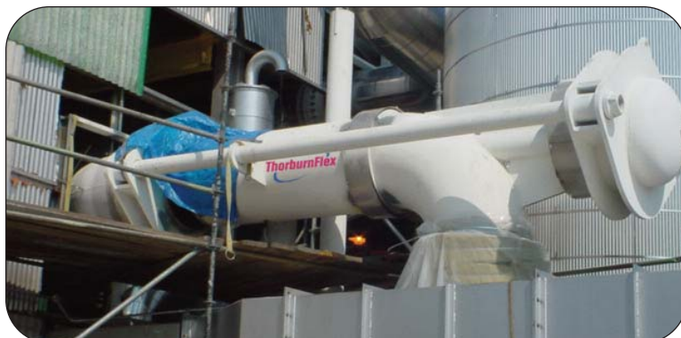
Thorburn crossover pressure balanced expansion joint installation
