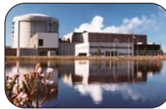
Clean Power Generation
