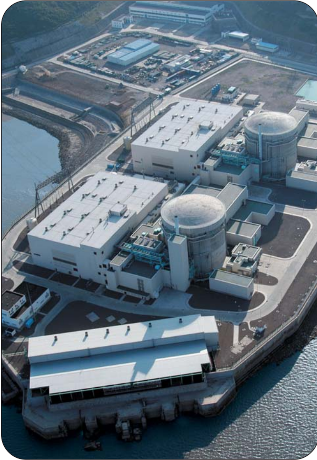
PHWR nuclear power plant in Qinshan, Haiyan County, Jiaxing, Zhejiang province, China
