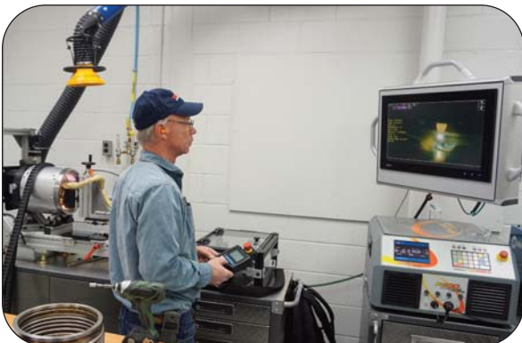
Thorburn's welding operator monitoring the automatic circumferential weld through a remote video camera
