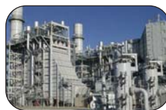
Clean Gas Power Generation
