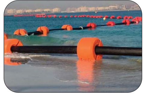
Dewatering and Dredging
