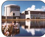
Clean Power Generation
