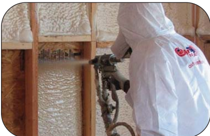
Insulation foam spraying
