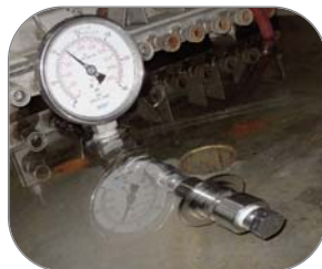
Pneumatic test at 100 psi
