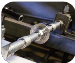
Hydrostatic test at 4000 psi
