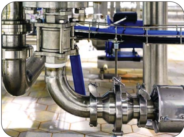
Sanitary flange clamp fitting installed
