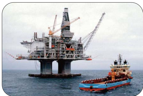
Hibernia offshore developmental project used Thorburn's flexible piping technology to provide external pressure containment, stress and movement absorption on its permanent ballast water containment piping system over 80 meters under the Atlantic Ocean, off the East coast of Newfoundland
