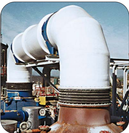
Quantity of 12 Thorburn 62HPW 900mm (36") Rubber Expansion Joints installed on a GRP piping system at a sulphuric acid plant in Baja Mexico
