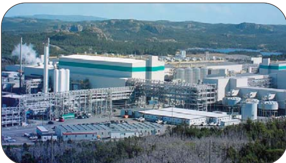
Thorburn was awarded the rubber expansion joint contract for the Vale Long Harbour, Nfld., Canada hydrometallurgical nickel plant
