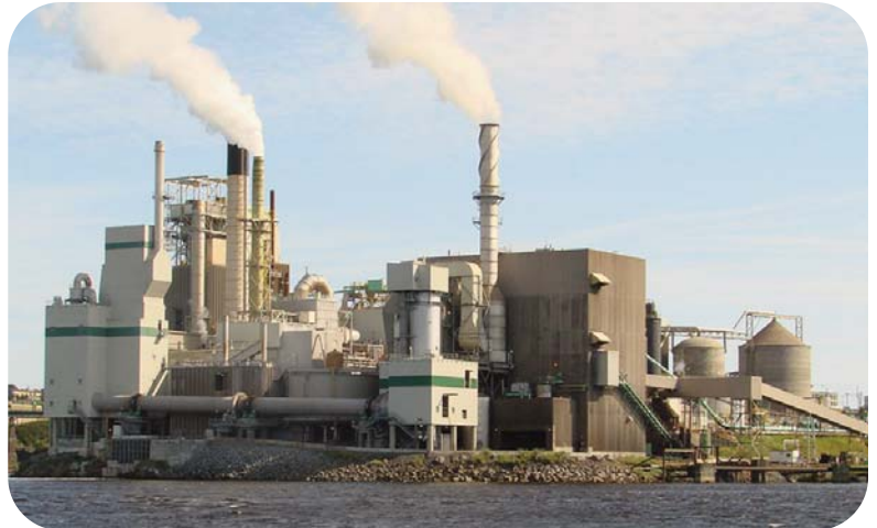
Irving Pulp And Paper Mill is situated on the St. John River at Reversing Falls uses Thorburn's flexible piping
