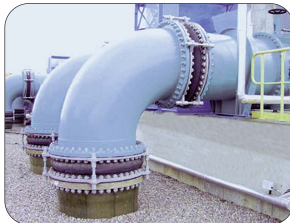
Thorburn's 42HPW 900mm (36") single arch rubber expansion joint with control rod system
