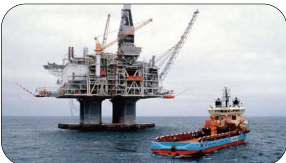
Thorburn was awarded the rubber expansion joint contract for the hibernia offshore oil rig in Newfoundland, Canada
