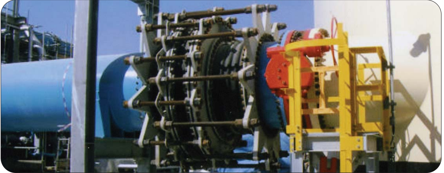
Thorburn's 42HPX-PB 1830mm (72") In-line Pressure Balanced Expansion Joint installed at a power plant in Saudi Arabia
