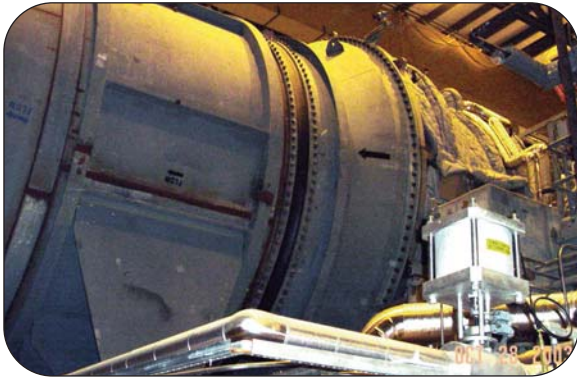
Thorburn's Dog-Bone expansion joint installed in a power plant in upstate New York, USA
