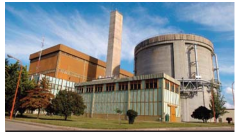
Clean Power Generation
