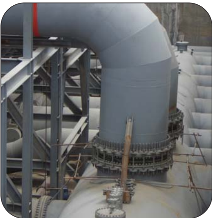
Quantity of 36 Thorburn 42HPW 1200mm (48") rubber expansion joints installed at a power plant in Iran
