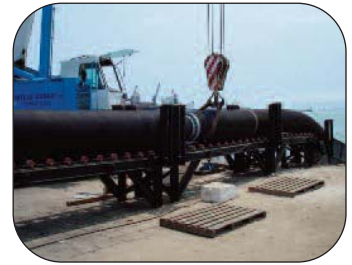
Sand & Gravel Dredging
