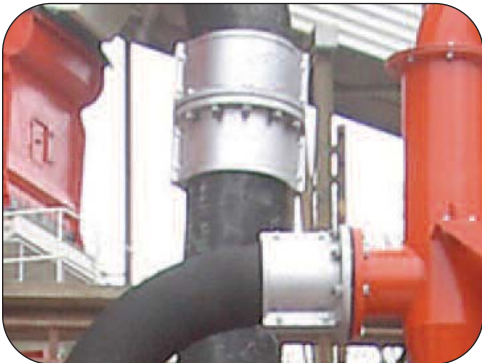
60TMH Split Cast Coupling Hose Assembly
