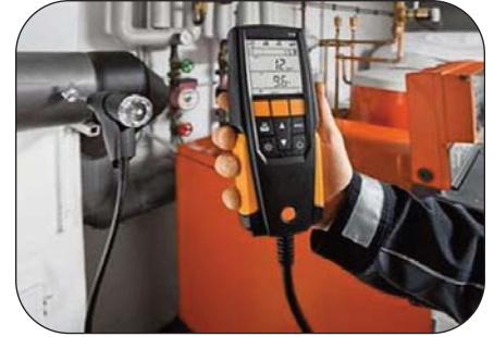
Flue gas analysis
