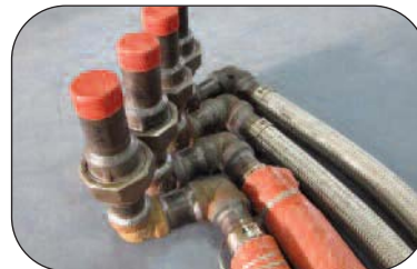
Flexible Piping Systems with Rigid Piping Connections
