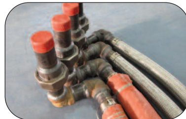
Flexible Piping Systems with Rigid Piping Connections
