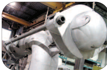
Pressure balanced crossover expansion joints
