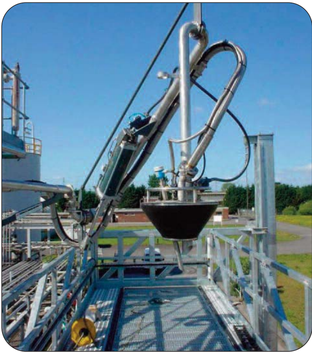
Chlorine Loading Platform
