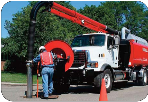
Sewer cleaning service
