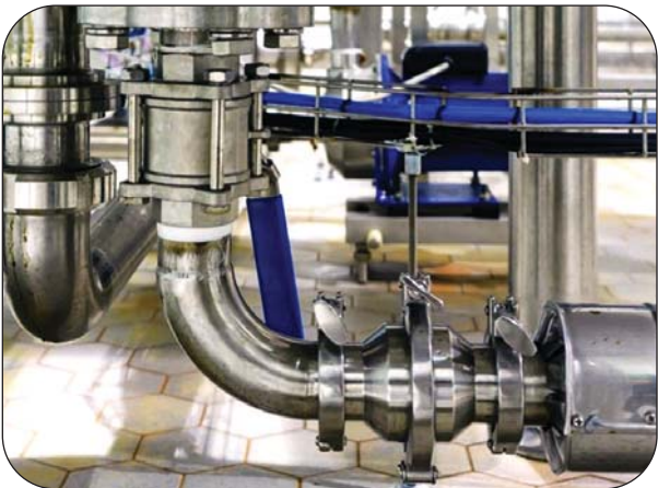
Sanitary flange clamp fitting installed
