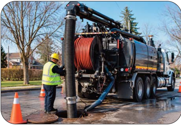
Municipal Sewer Cleaning
