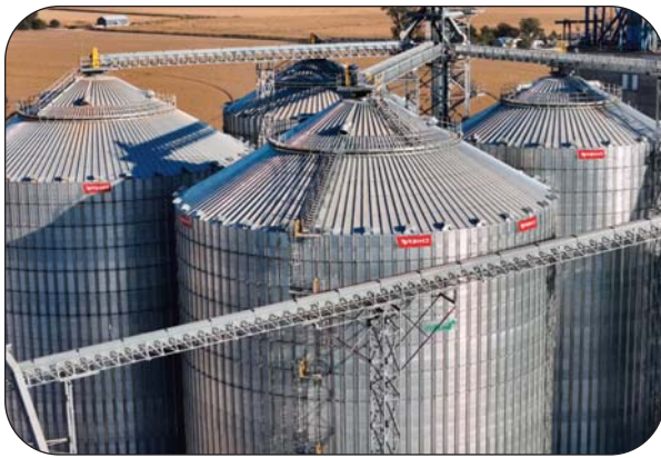
Silo Grain Conveying Systems
