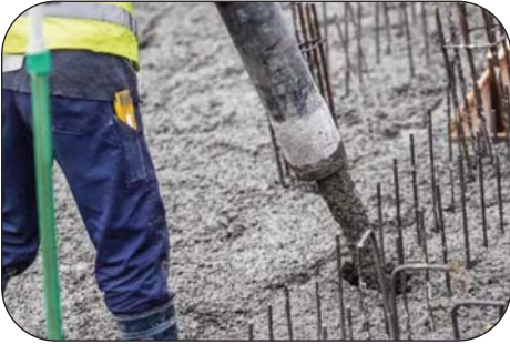
Concrete Placement and Aggregate Handling
