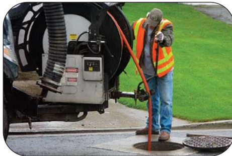
Commercial Sewer Cleaning
