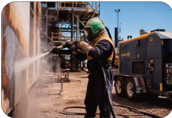
Mobile blasting equipment service
