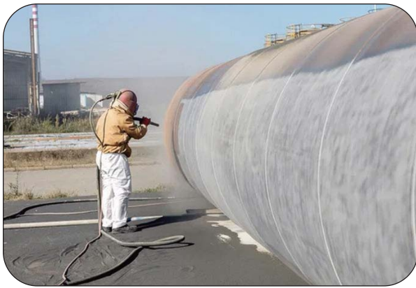
Sandblasting Metal Spool Pipe
