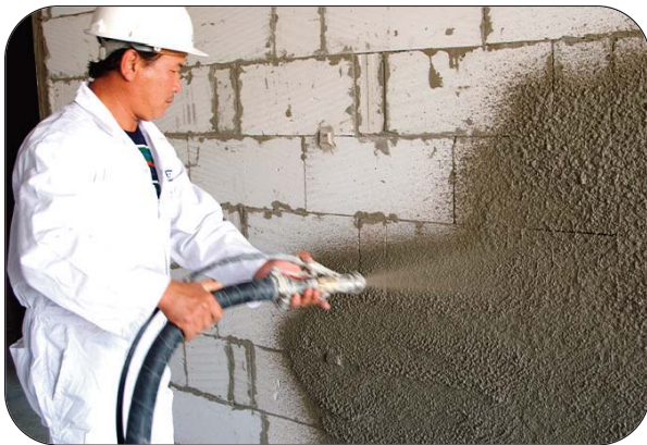
Cement spray placement
