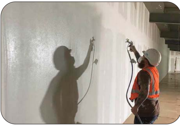
Plaster spray placement
