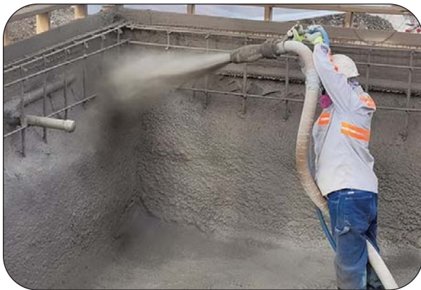
Guniting spray placement
