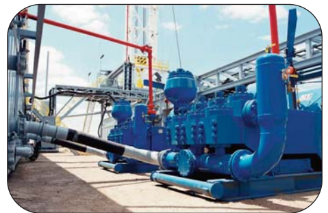
Mud Pump Discharge Lines
