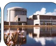
Clean Power Generation
