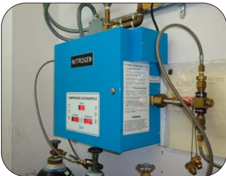
Pigtail hoses on nitrogen gas manifold
