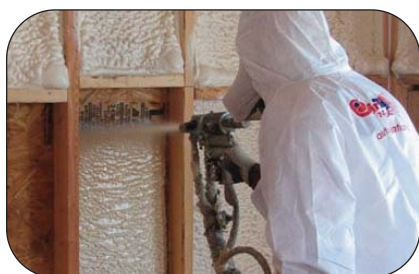
Insulation foam spraying
