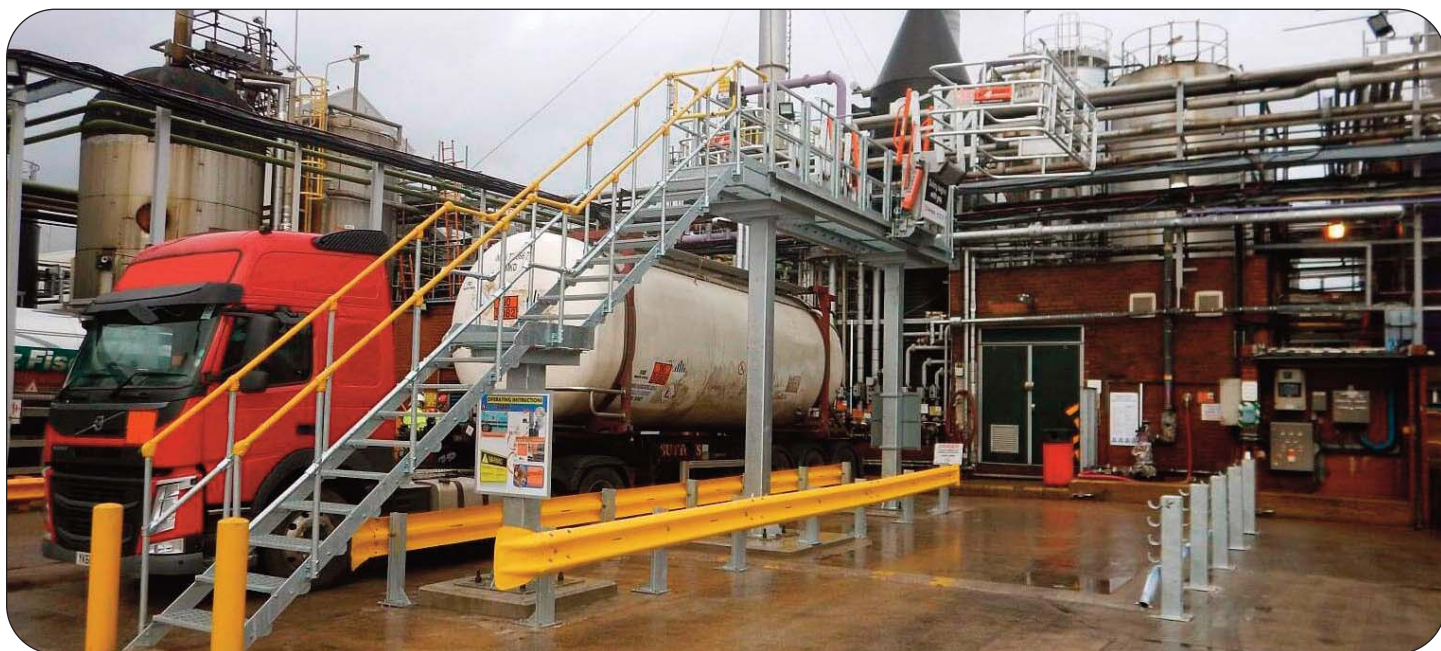
Chlorine Unloading Station
