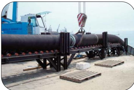
Sand & Gravel Dredging
