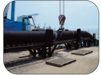
Sand & Gravel Dredging
