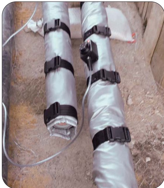
Thorburn's ThermaCover™ Series TCT-HT removable insulation jacket with integral heat tracing elements
