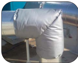
Elbow Pipe Design
